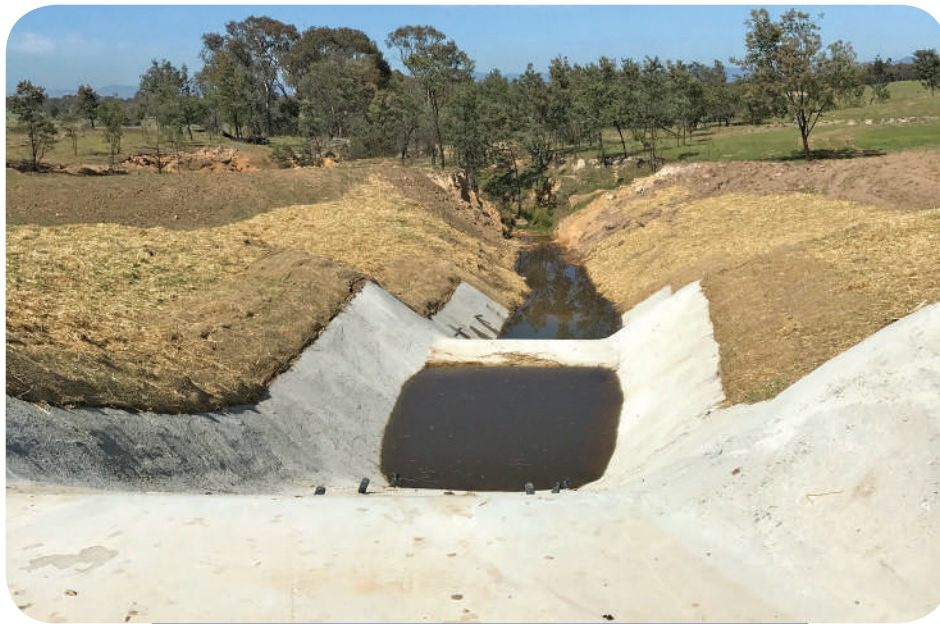
Concrete flume: directing flow into stilling pond.
