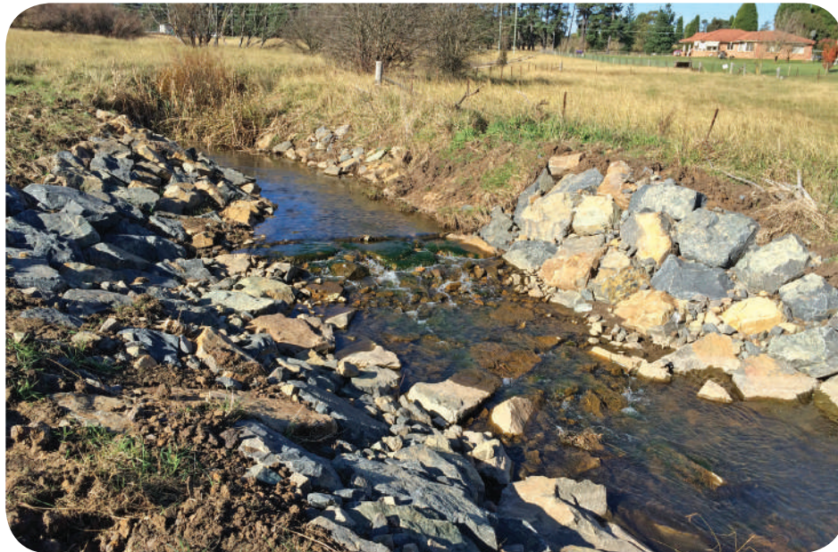
Grade Stabilisation Structure
