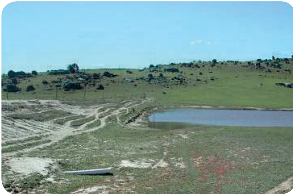
Pipe through bank of gully control structure (dam) to reduce the frequency of flow through primary spillway. This helps to prevent the spillway becoming sodden and prone to erosion.
