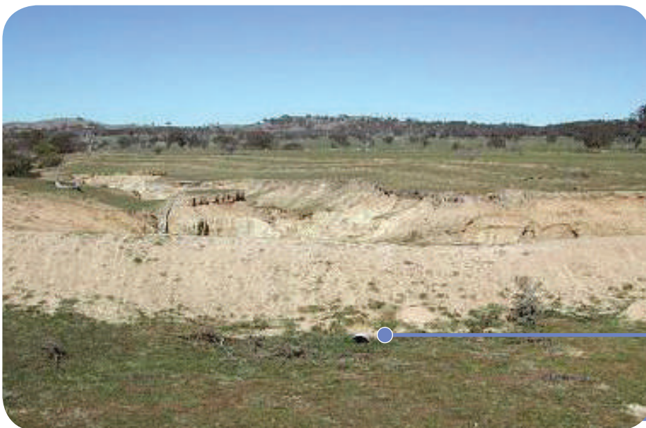
Pipe through diversion bank protecting gully head below.
