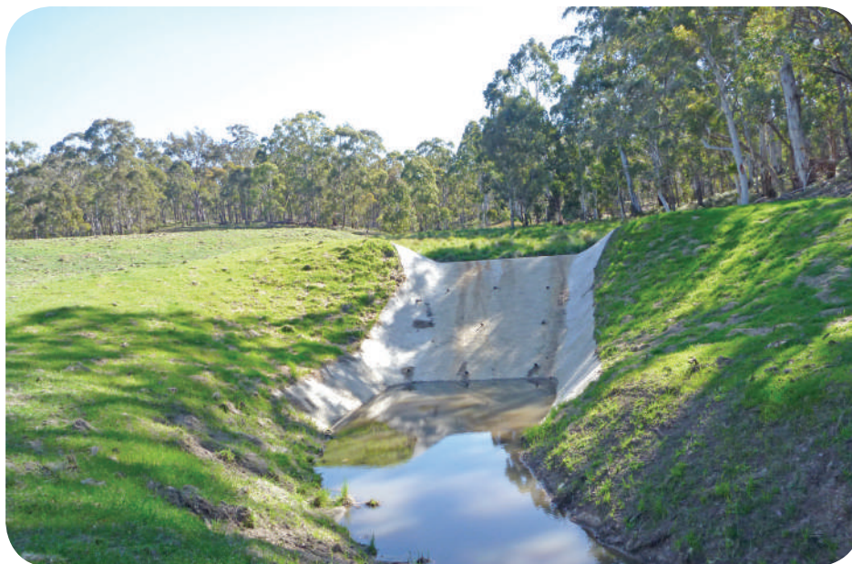
Concrete flume well vegetated.
