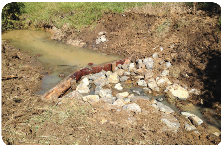
V Notch Weir
