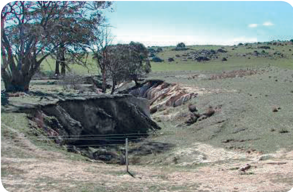
View of gully below gully control structure.
