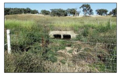
The culvert showing washed out soil
