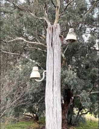
A timber pole used to carry a telephone line
